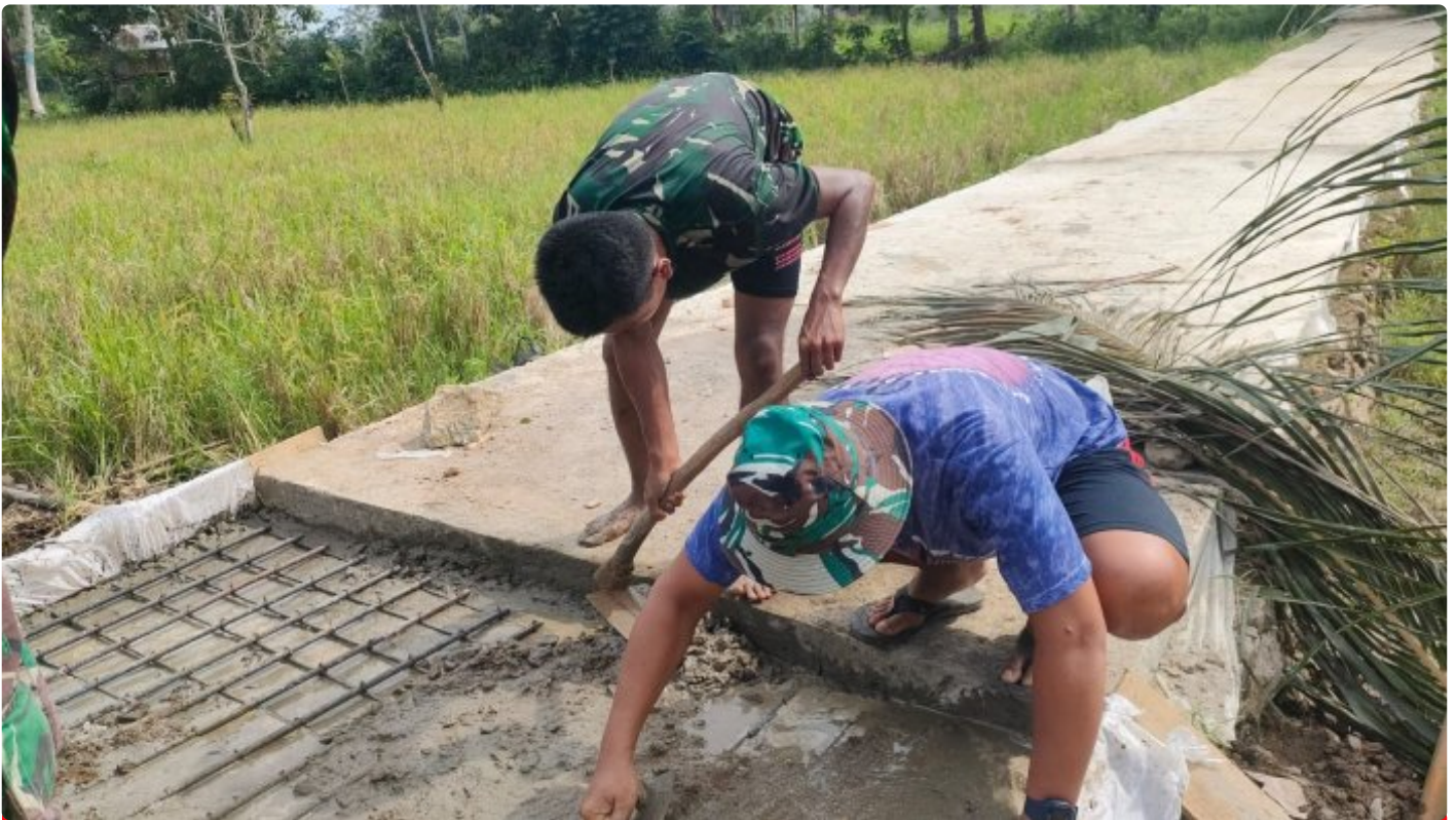
Slop Beton 1 Sasaran TMMD 116 Kodim 1002/HST Capai 60 Persen
